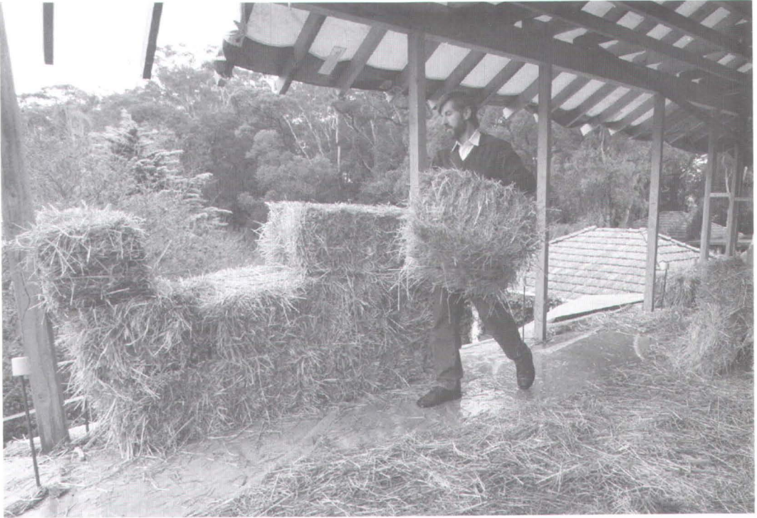
The second storey of a Killara home being built with straw — the building process is undergoing accreditation by Ku-ring-gai Council.
